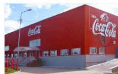
Coca Cola Plant Project (South America)
