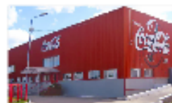
Coca Cola Plant Project (South America)
