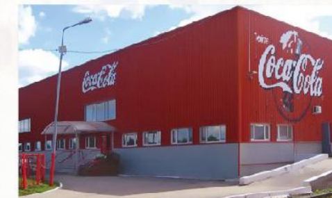
Coca Cola Plant Project (South America)
