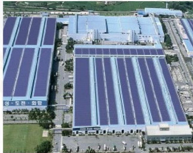
Renault-Samsung Busan Sola generating parking lot construction
