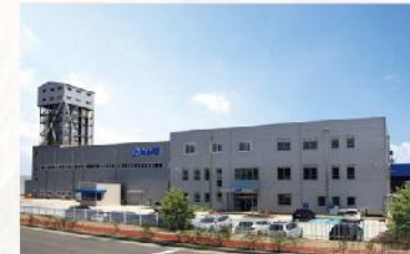
Mapei Cheonan factory construction
