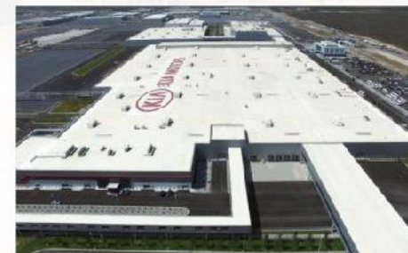
Kia Mobis India factory construction (India)
