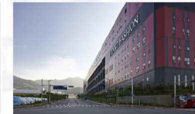
Cheonan E-Land Logistics Center construction
