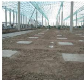
| Pile Ground Reinforcement
