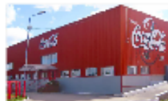
Coca Cola Plant Project (South America)
